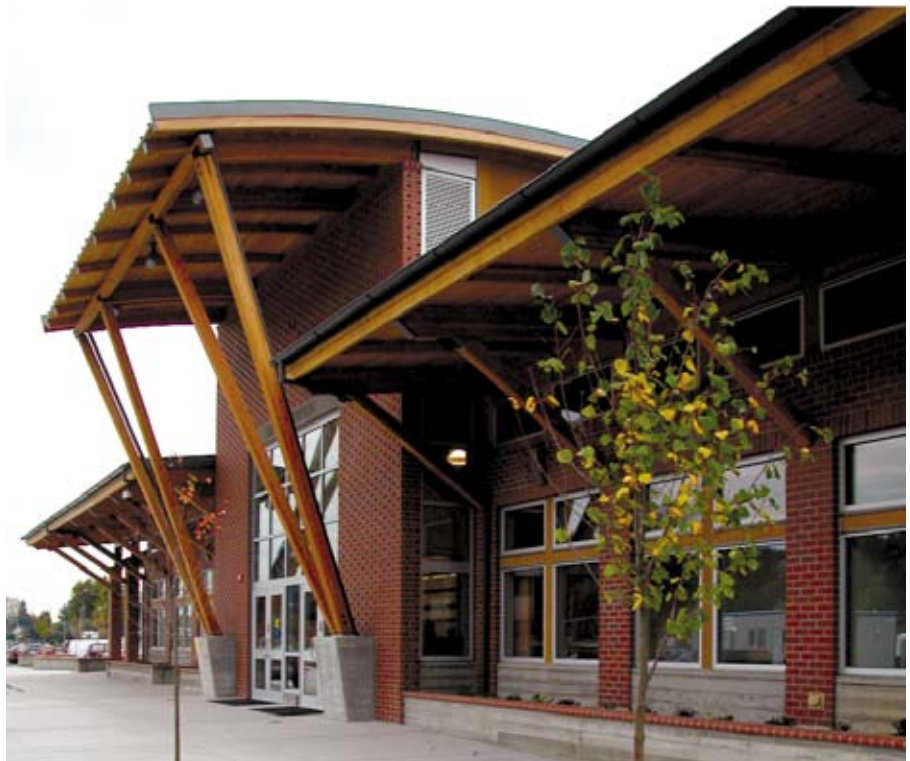
The architect of the Skagit Station juxtaposed glulam with brick to help the new structure fit into the historic community.
