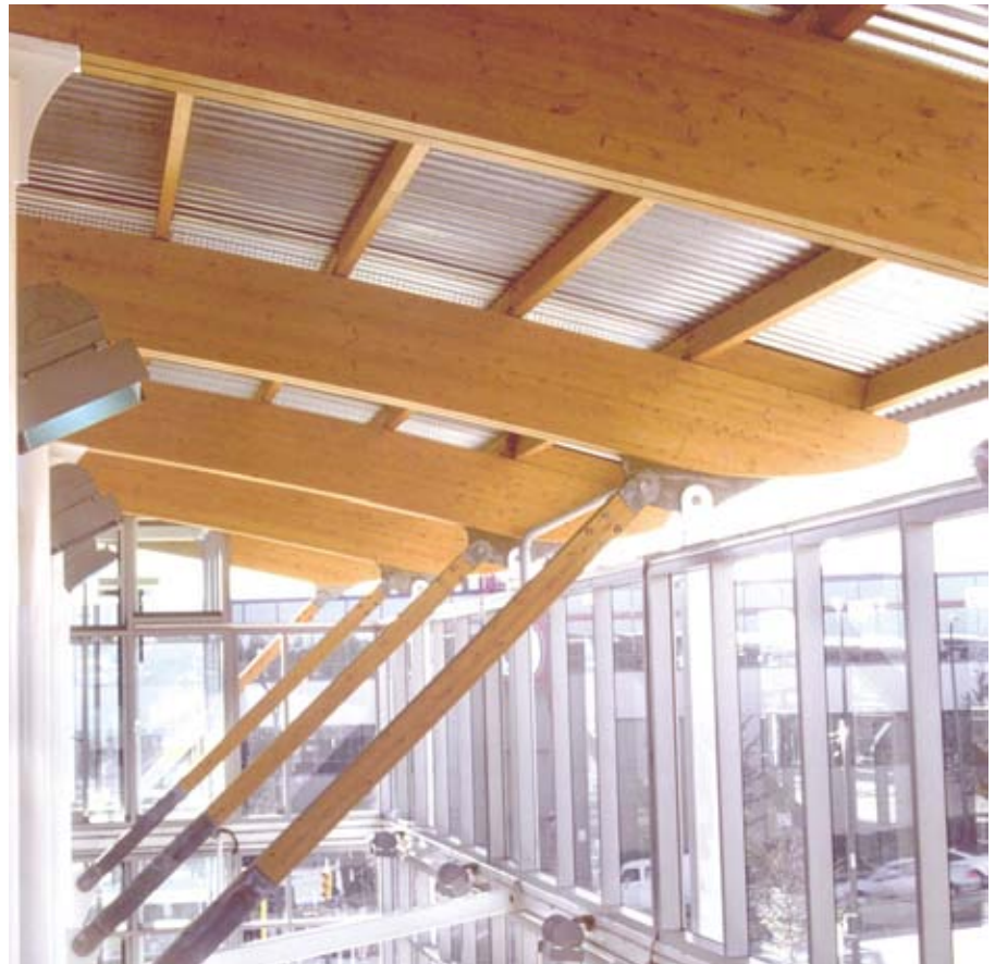
Architects used glass and a modern, open concept that incorporates the principle of "see-in, see-out," while glulam creates a station that is warm and welcoming.
