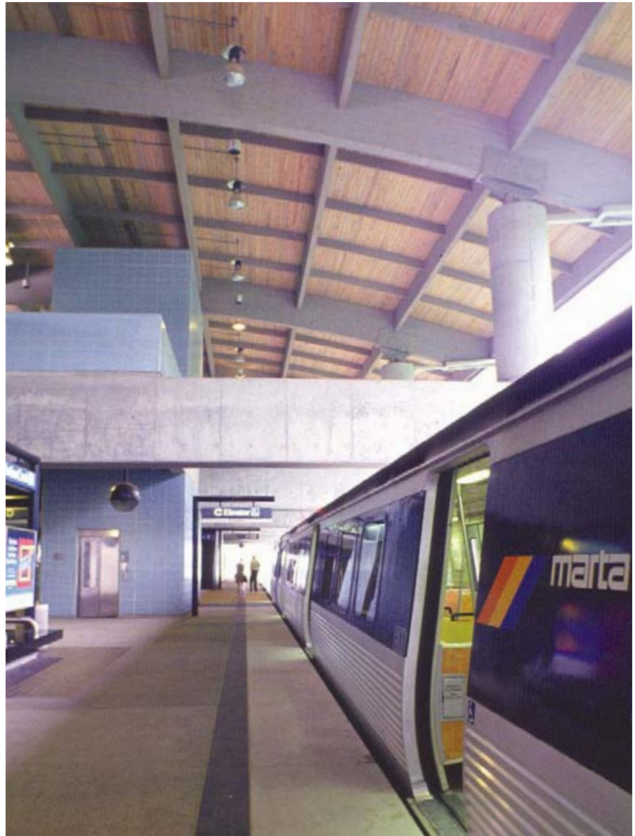
Indian Creek Station in Atlanta features 14 curved glulam girders spaced 40 feet apart, forming a barrel vault with a 180-foot radius.
