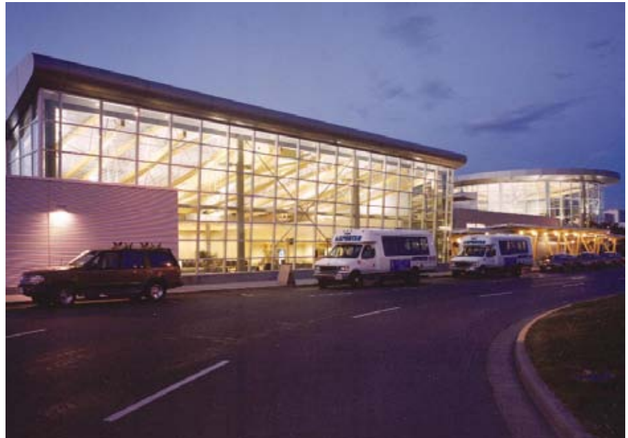
Spruce glulam trusses helped architects achieve the desired look and keep construction on budget.
