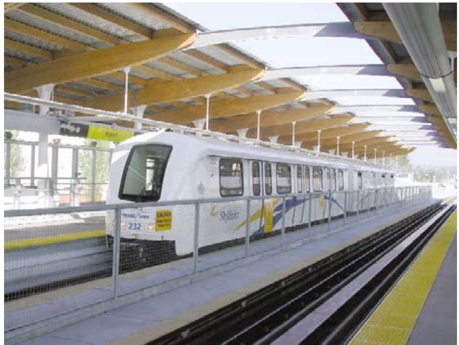
When glulam is left exposed yet protected from the elements, as it was for the Rupert Station in Vancouver, BC, the structure can stand 100 years or more.
