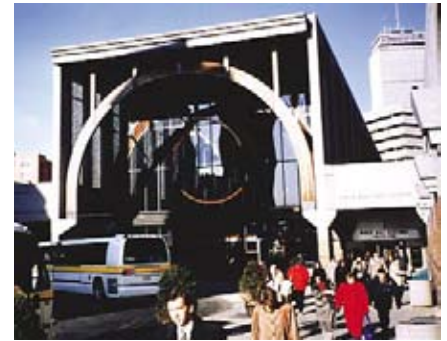
Large stained glass windows were used at each end of the Back Bay station to provide additional natural lighting for thousands of Boston's daily commuters.
