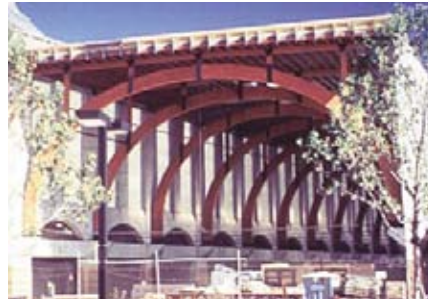
The 18 pairs of glulam radial arches used in the Back Bay Station span approximately 65 feet, creating an eye-catching wooden structure in downtown Boston.
