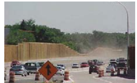
Sound barriers made from glulam fit well within residential neighborhoods while providing strength, durability and low cost.
