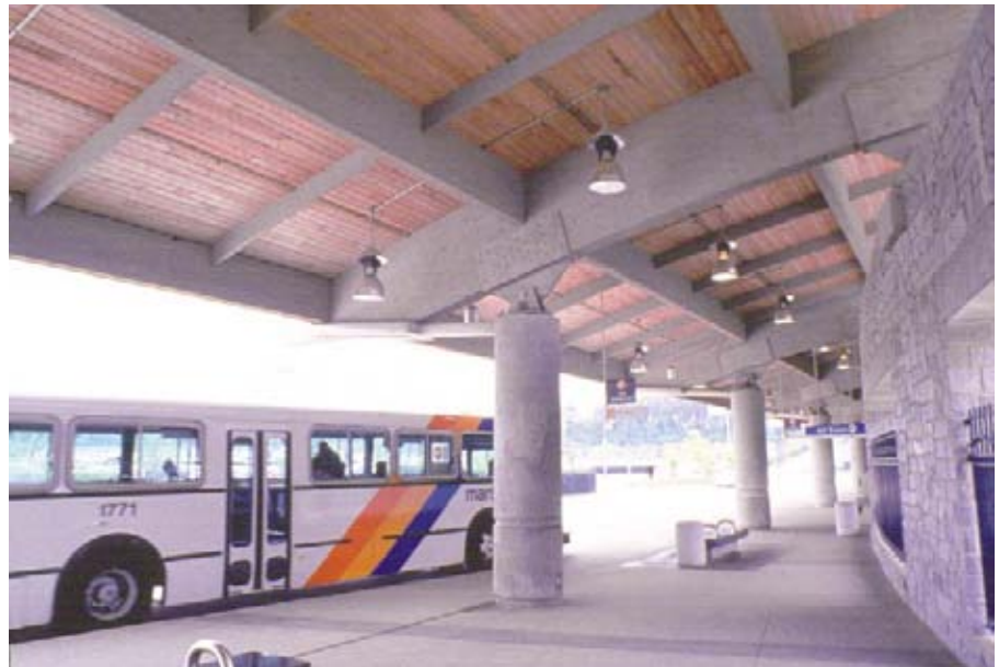
The wood roof structure of MARTA's Indian Creek Station weighed less than comparable steel or concrete systems, allowing architects to use smaller support columns, which reduced the cost of the foundation.
