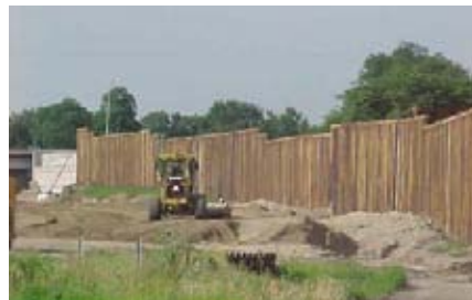
Sound barriers made from glulam fit well within residential neighborhoods while providing strength, durability and low cost.
