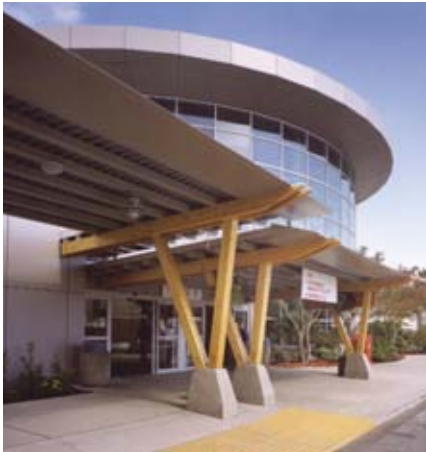
Covered walkways are designed with glulam to warmly welcome passengers to the Victoria Air Terminal.
